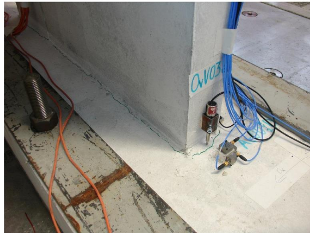
Figure 21: Crack at the bottom of wall 04 after Northridge 0.40g (DEN, 2014)
